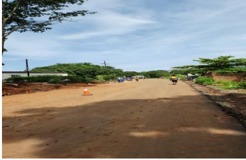
UPGRADING OF NDOLA ROAD
