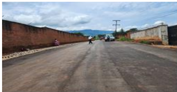
UPGRADING OF KALIMBUKA ROAD
