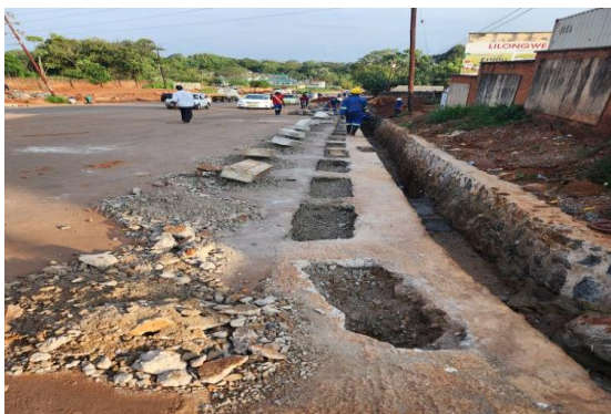
UPGRADING OF NAMIWAWA DUALISATION
